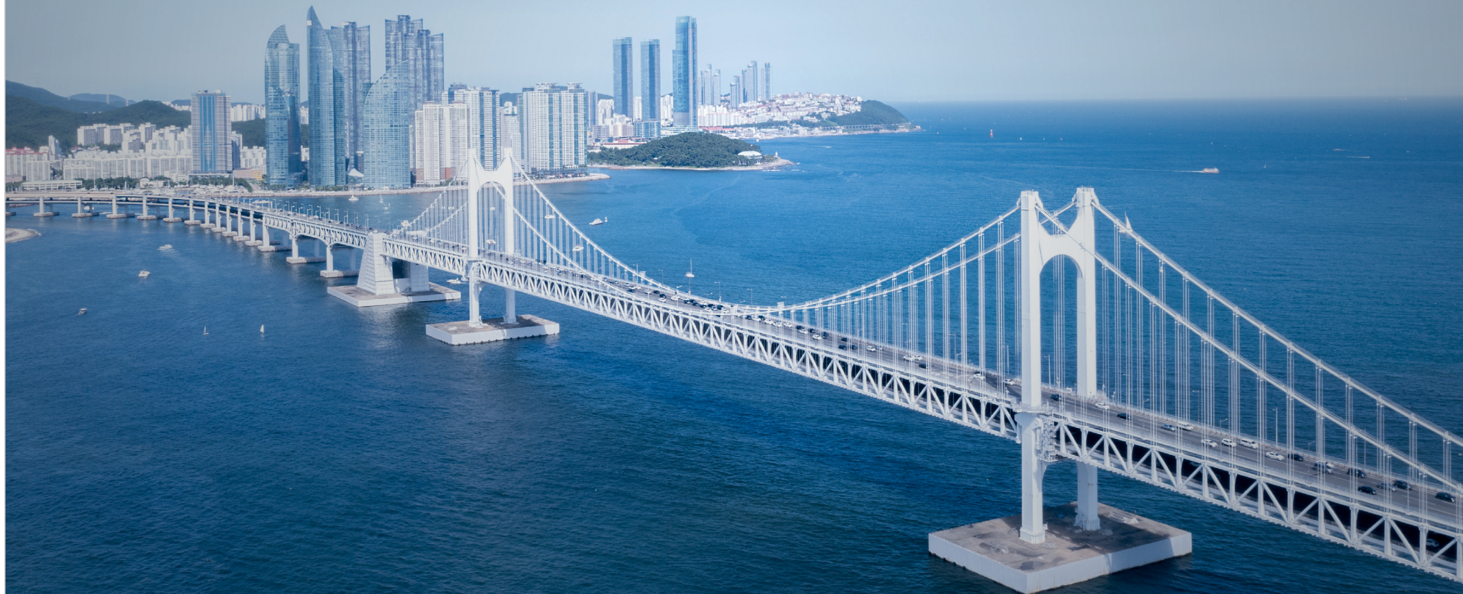
Full View of Gwangan Bridge in Busan
